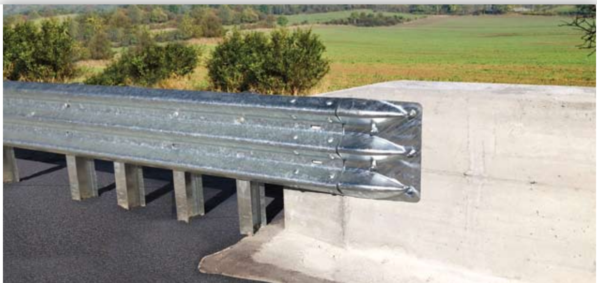
Figure 4: Structural connector to concrete
