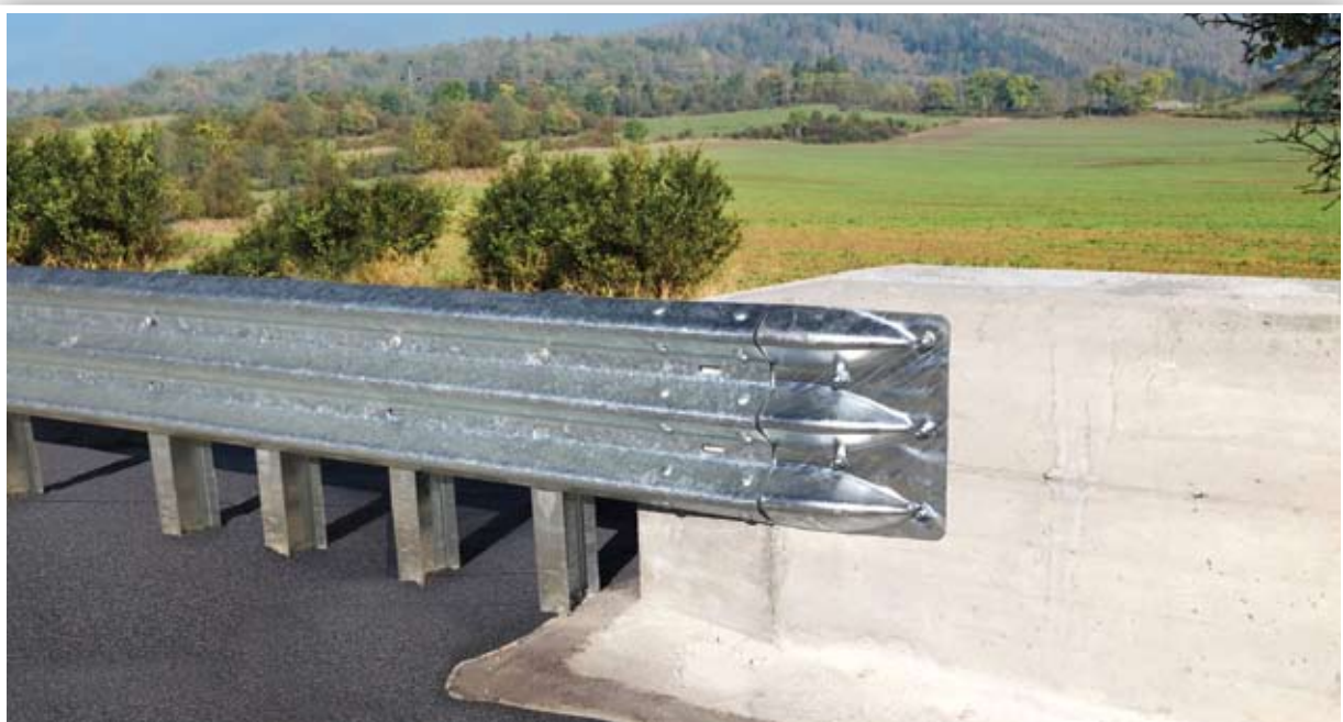
Figure 4: Structural connector to concrete
