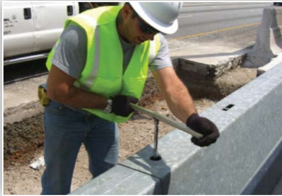
Security Nut Installation
