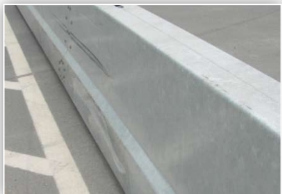
Typical Impact Damage
