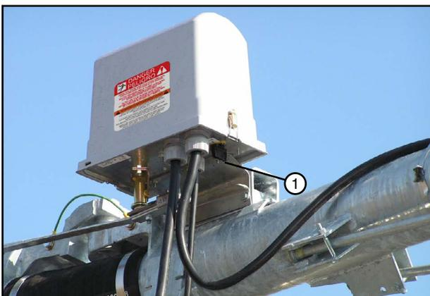
Figure 12-1 1. Disconnect Switch
