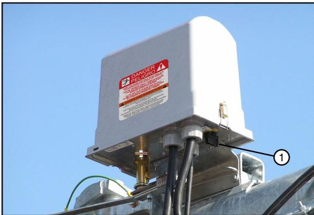
Figure 12-1 1. Disconnect Switch
