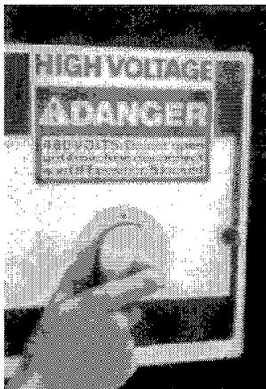
Turn **DISCONNECT SWITCH** to "ON". If power is supplied by engine driven generator, adjust RPM until **VOLTMETER** reads 480 volts to 505 volts.
