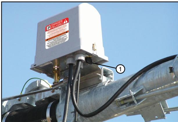
Figure 12-1 1. Disconnect Switch
