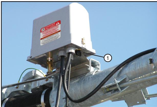
Figure 14-1 1. Disconnect Switch
