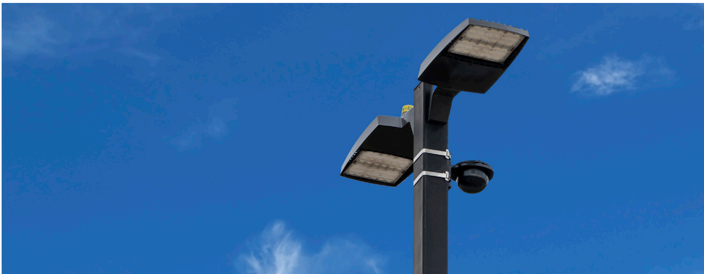
The Valmont Mitigator LP3 Vibration Damper Mounted to Square Light Pole
