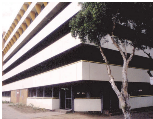
Old made new. All security mesh panels on lower level were re-galvanized and returned to service.
