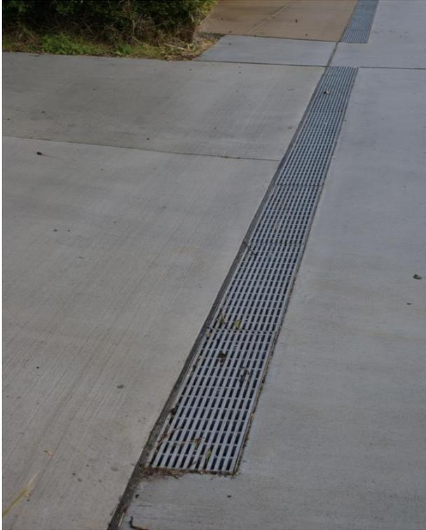
These photos show our 200mm clear opening drainage channels complete with locked down longitudinal heelguard grates after installation.
